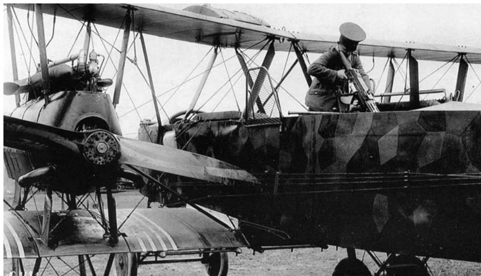
TOP: Flown by a three-man crew, the two-engine Gotha G.V. heavy bomber could carry as many as ten 110 lbs. bombs. The Germans conducted 52 airstrikes on Great Britain using Gotha and "Giant" bombers. BELOW: A German gunner demonstrates how the Gotha's 7.92mm dorsal machine gun on a pivoted mount could be fired down through the fuselage.
