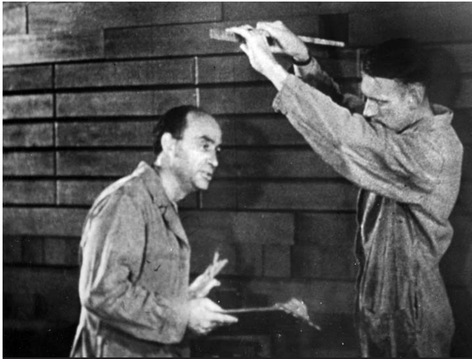
ABOVE: Scientist Enrico Fermi (left) and an assistant examine the venier control rod that would be slowly removed from the radioactive pile to increase the rate of nuclear fission in the historic chain reaction. BELOW: Chicago Pile-1, consisting of blocks of graphite containing uranium oxide, is shown under construction at the University of Chicago. Intended to help prevent the loss of neutrons, the Goodyear balloon cloth draping shown at left and to the rear proved unnecessary during the process that generated the historic nuclear chain reaction.
