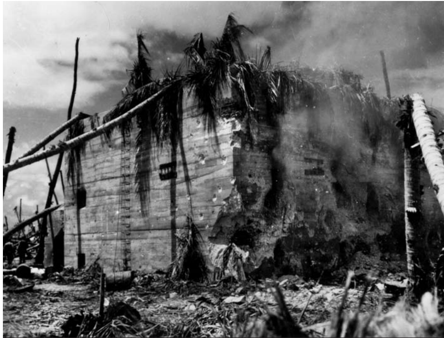
The Japanese command bunker on Tarawa was built of reinforced steel and concrete. Commander Keiji Shibasaki, and most of his staff were killed by a navy shell as they were exiting the bunker on the first day of the invasion.
