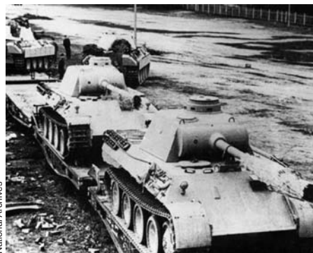
RIGHT: The Mark V Panther medium tank was the German response to the outstanding performance of the Red Army’s T-34. The Panther sported sloped hull armor and a 75mm high velocity cannon.
