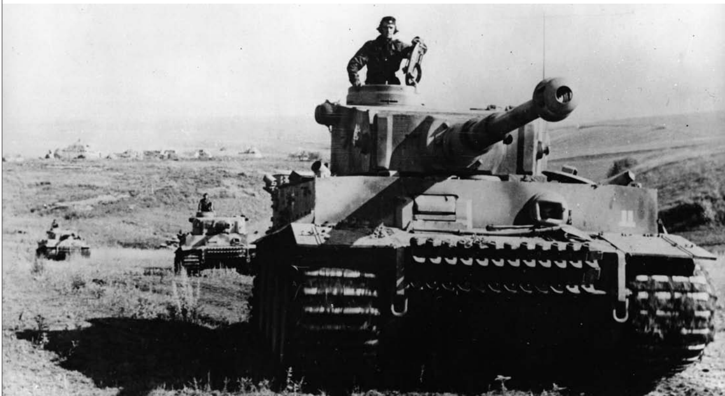
The Mark VI Tiger tank, with its 88mm cannon, was perhaps the most feared weapon in the Wehrmacht arsenal; however, the mammoth tank was plagued by mechanical failures and an insatiable appetite for fuel.
