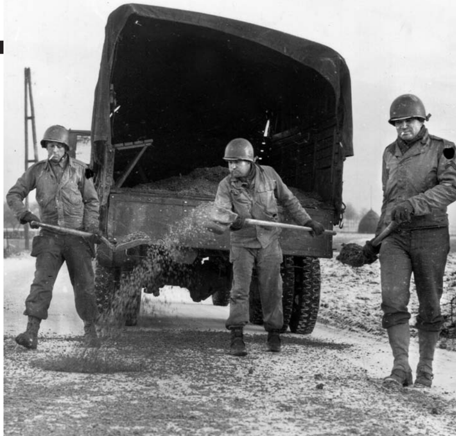
ABOVE: U.S. Army combat engineers shovel cinders onto an icy road in Belgium during the Battle of the Bulge. This effort was essential in moving Allied troops forward in response to the German thrust through the Ardennes Forest during December, 1944, into January, 1945. OPPOSITE: A German Fallschirmjäger hands a cigarette to a messenger who has just come up on a motorcycle during the advance of the 501st Heavy SS Battalion in the Battle of the Bulge. The German paratroopers pictured aboard the Tiger tank were attached to Kampfgruppe Peiper. The German battle group led by SS Lt. Col. Joachim Peiper was intent on capturing bridges at Trois-Ponts, Belgium, but heroic American combat engineers thwarted his plan.
