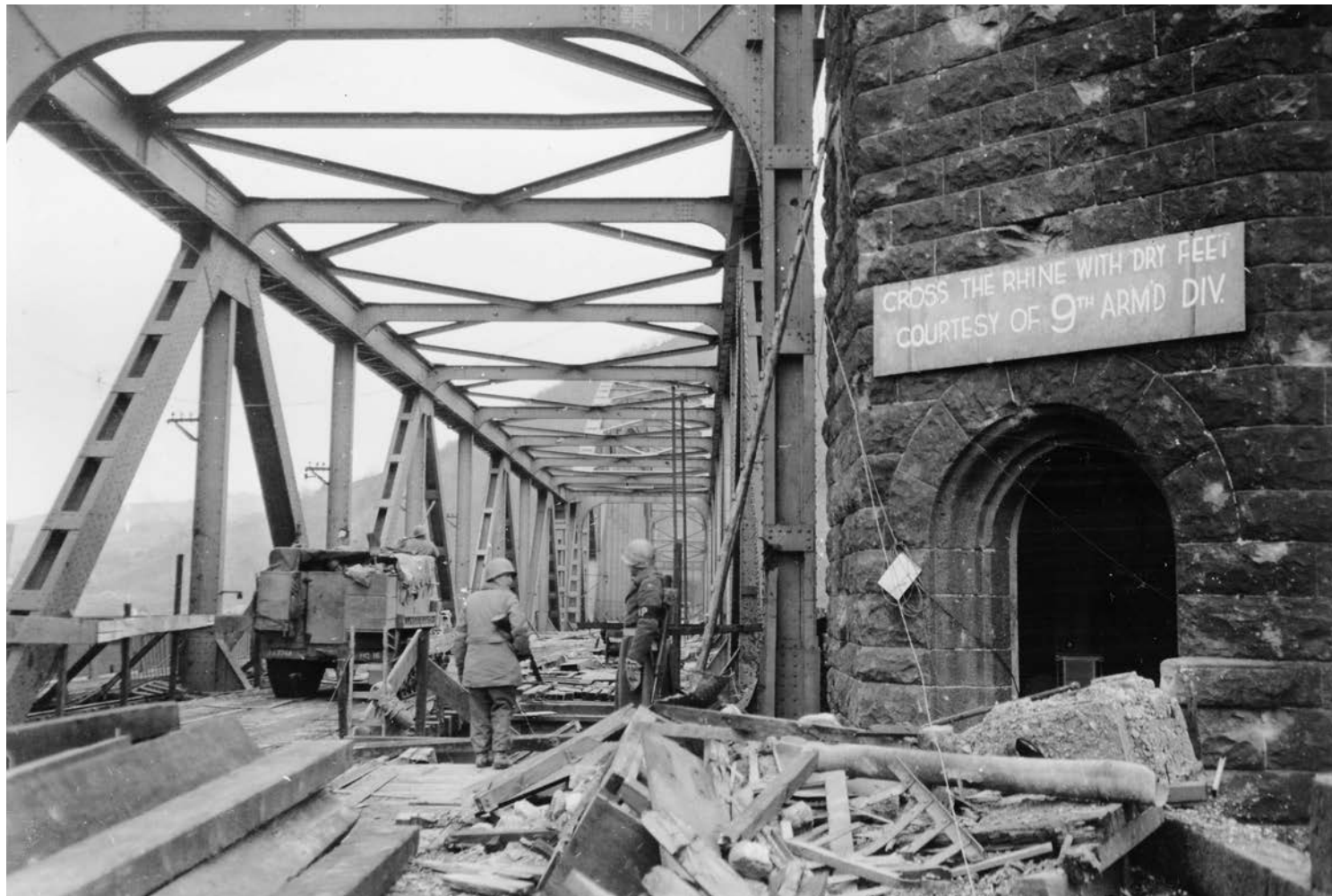
U.S. forces cross the Ludendorff railroad bridge at Remagen on March 8, 1945. Combat engineers had cleared debris from the German's failed effort to blow the bridge the day before and installed wooden decking. Until it finally collapsed on March 17, the Germans attacked the bridge with infantry and armor, howitzers, mortars, floating mines, mined boats, a railroad gun, and more than 300 aircraft.
