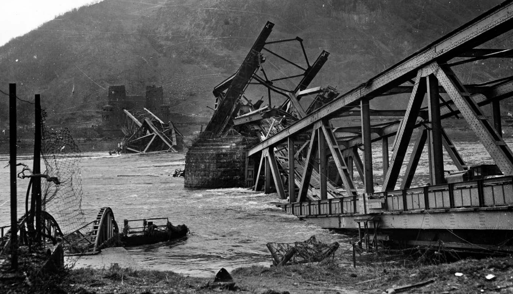
ABOVE: American engineers attempted to shore up the Ludendorff bridge while pushing across as many troops as possible. Attacks by German aircraft and V-2 rockets, in addition to the damage from the initial demolition attempt, finally caused the bridge to collapse on March 17. Six soldiers from the 276th Engineer Combat Battalion died; 11 were missing and presumed drowned; 60 were injured, and three later succumbed to their injuries. OPPOSITE: A U.S. antiaircraft battery guards a pontoon bridge built by the 291st Engineer Combat Battalion (ECB). When weather cleared the Germans sent waves of aircraft to bomb the bridge, including Stukas and the jet-powered Ar-234, and the Me-262. Twenty-six aircraft were shot down over the course of two days, with more damaged.
