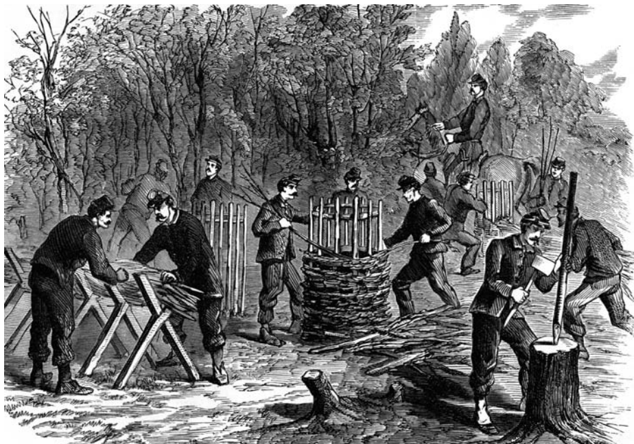
Men of the 77th Pennsylvania Regiment construct fascines and gabions for breastworks.
