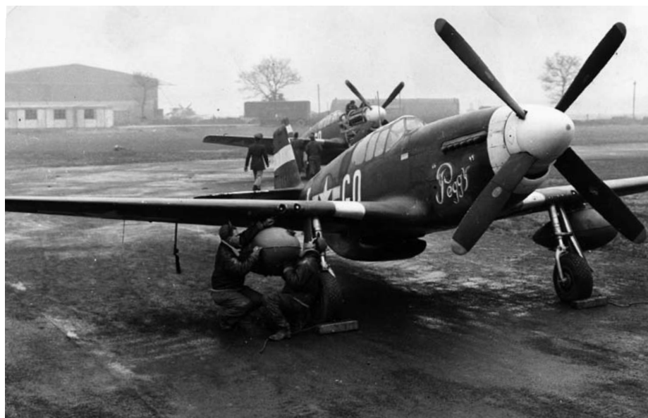
ABOVE: On a muddy airfield in England, P-51 Mustangs sit ready for their pilots to climb aboard as two ground crewmen make a final check of an external drop tank. The extra range provided by the drop tanks allowed the fighters to escort bomber formations deeper into Germany. RIGHT: During a fighter bomber mission, Lieutenant Colonel Wallace Hopkins of 8th Fighter Command releases his bomb load from his P-51 Mustang nicknamed "Ferocious Frankie." The Mustang proved capable in both the escort and ground attack roles.
