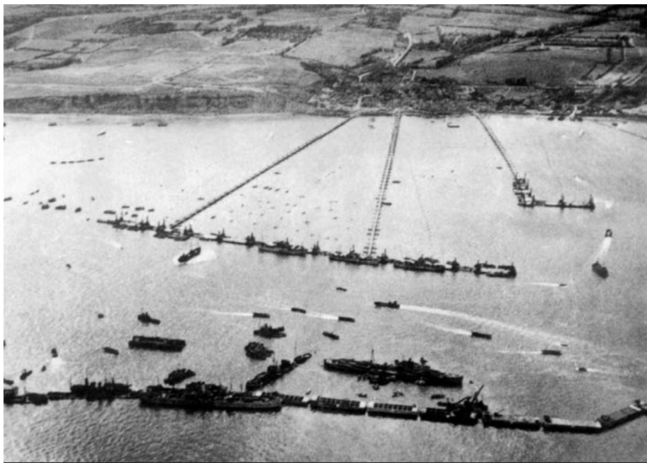
Shown deployed along a Normandy invasion beach, this Mulberry artificial harbor allowed supplies and reinforcements to be offloaded in support of the Allied landings which took place on June 6, 1944. This aerial view provides a perspective of the size of the massive structure. (Imperial War Museum)
