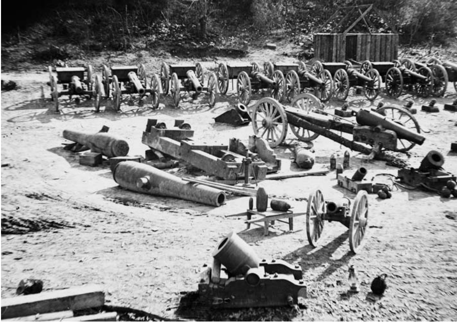
TOP: A drawing of the area south and east of Broadway Landing from the 180-foot-high Cobb's Signal Tower shows Point of Rocks Bridge, the town, and its pontoon bridge. ABOVE: This famous photo shows mortars and other large artillery pieces on the beach below the town.
