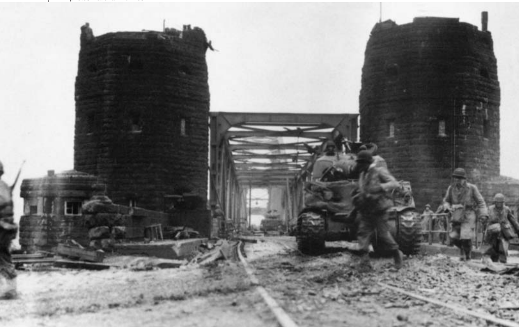
A column of American M4 tanks from the First Army rumbles across the bridge to establish a viable bridgehead east of the Rhine River.
