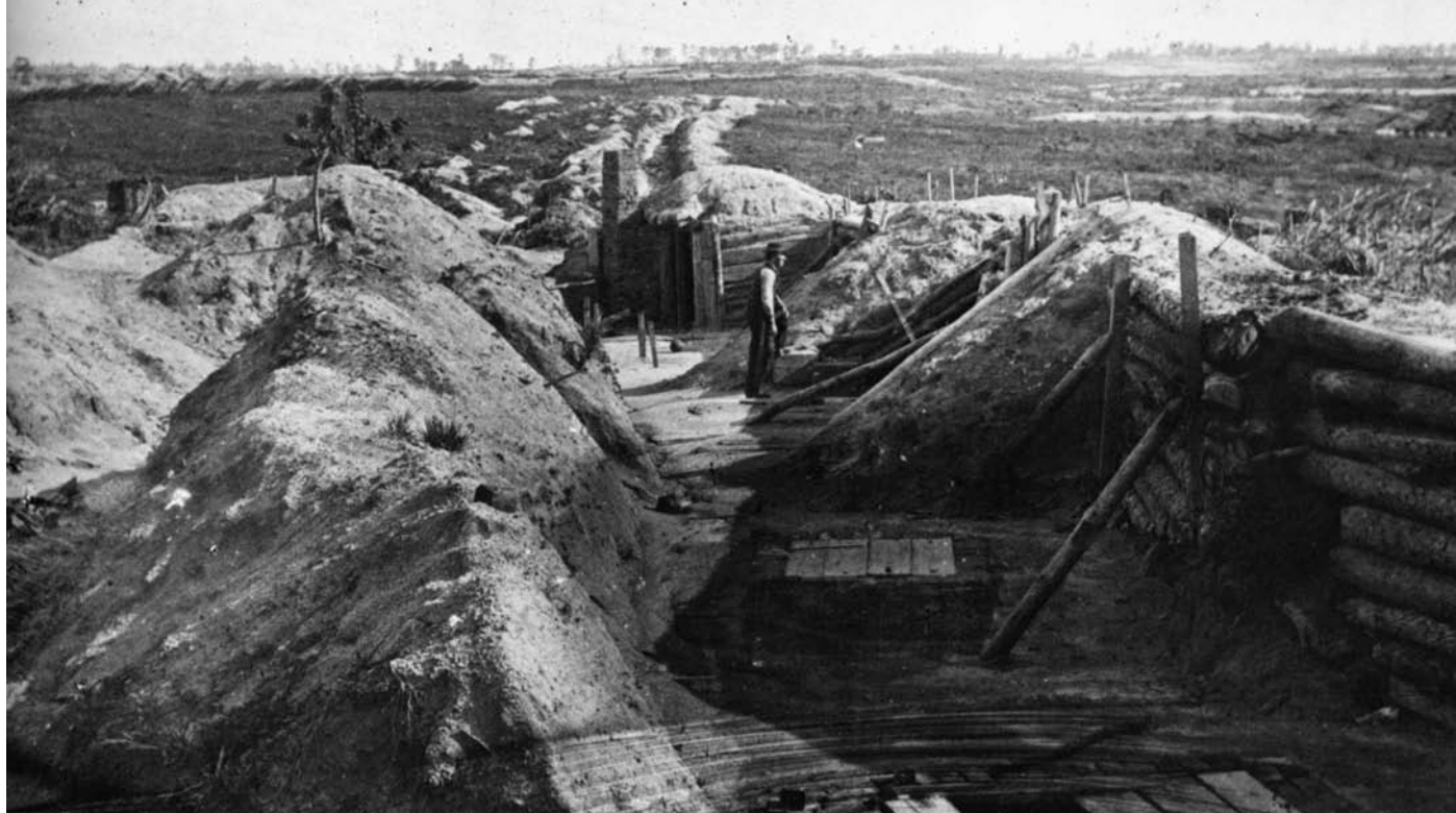
ABOVE: Deep trenches like this one, across from Elliott's Salient, helped conceal Union miners from Confederate eyes as they tunneled under enemy lines. LEFT: The tunnel Lt. Col. Henry Pleasants and his men dug ran for 510 feet.
