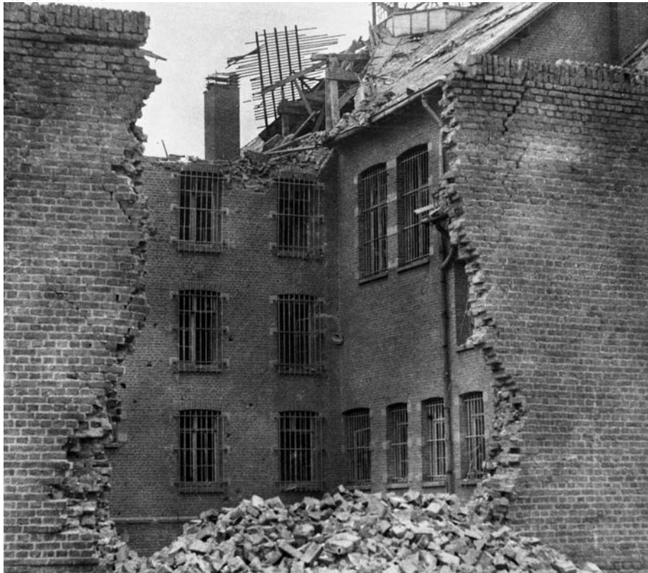
ABOVE: This photo, taken from inside Amiens Prison after the Operation Jericho raid, reveals serious damage to the complex. The junction of the north and west wings of the prison has been struck by several bombs. The photographer's back is to the large breach which was blasted in the outer west wall of the prison. OPPOSITE: Australian combat artist Dennis Adams captured the drama of Operation Jericho in Breaching of Amiens Prison as a Mosquito bomber rises from the complex, which is shrouded in smoke from bomb blasts.
