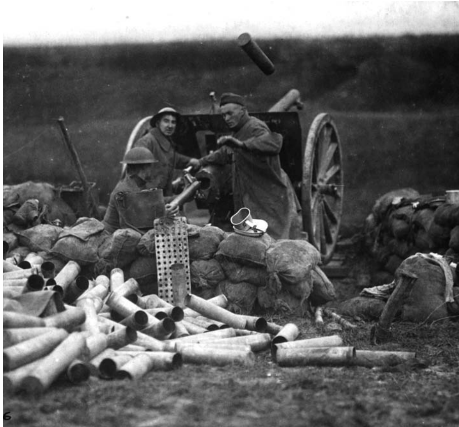
An American gun crew fires the 75mm at Saint-Michel, France, in September 1918. Note the large pile of expended shells and ammunition packing tubes behind the gun, indicating its high rate of fire. A shell casing is still in the air above the cannon.
