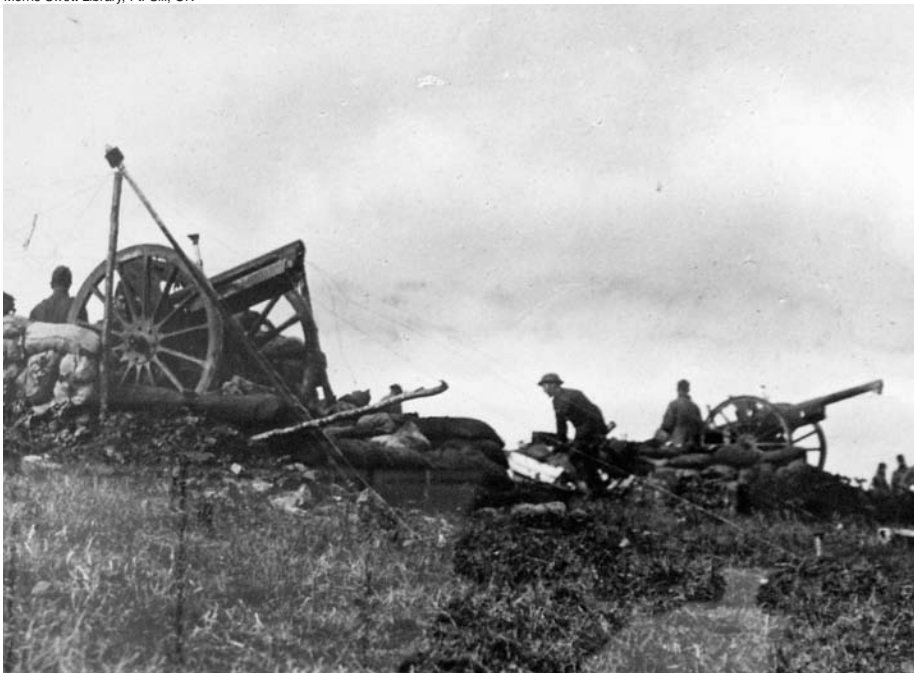
American doughboys handle a Model 1897 75mm in battle. The gun on the left is in full recoil, with a shell casing suspended in the air to the left of the tube.
