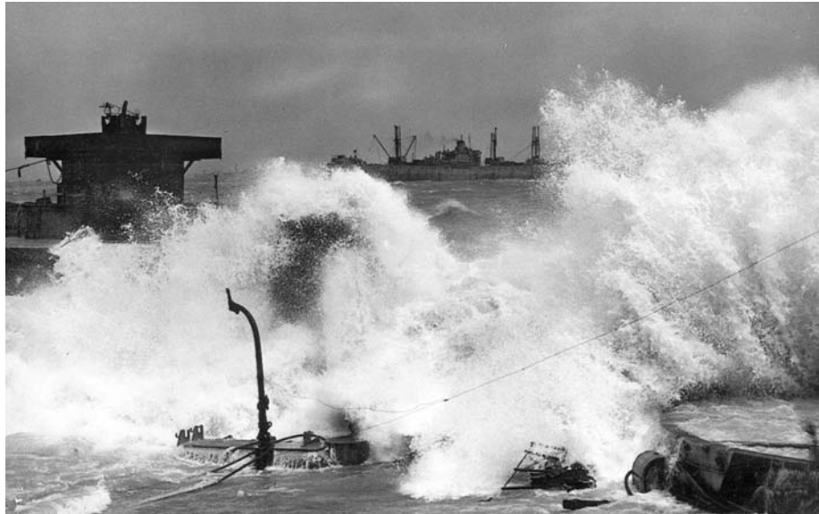
ABOVE: On the day after the successful Allied landings in Normandy, 23 old freighters were towed to the French coast and sunk bow to stern to form the outer breakwater of a Mulberry harbor. BELOW: In the wake of the savage storm that struck the Mulberries, small craft, vehicles, and components of the harbors themselves lie in shambles. One Mulberry was rendered completely useless by the violent weather.
