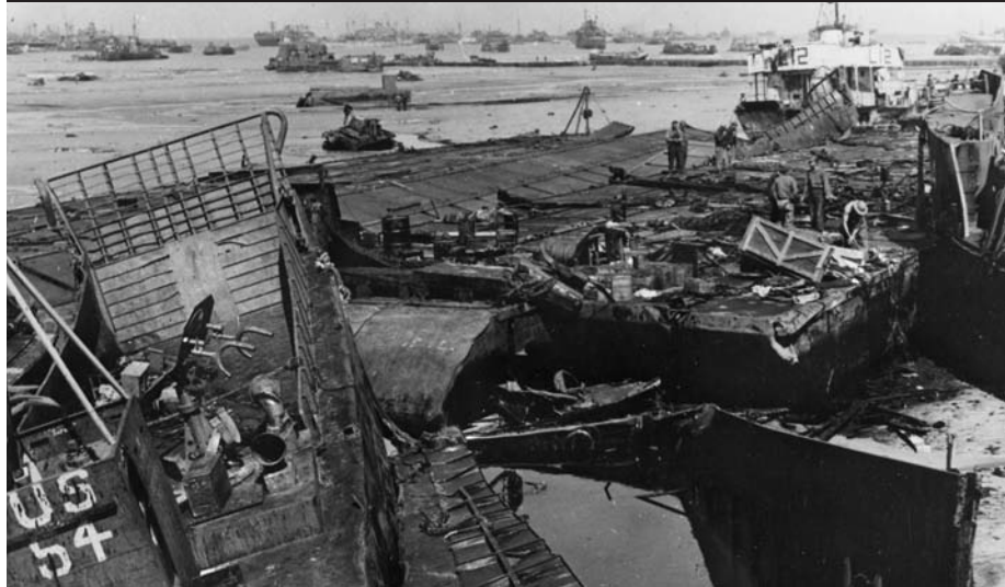
ABOVE: On the day after the successful Allied landings in Normandy, 23 old freighters were towed to the French coast and sunk bow to stern to form the outer breakwater of a Mulberry harbor. BELOW: In the wake of the savage storm that struck the Mulberries, small craft, vehicles, and components of the harbors themselves lie in shambles. One Mulberry was rendered completely useless by the violent weather.
