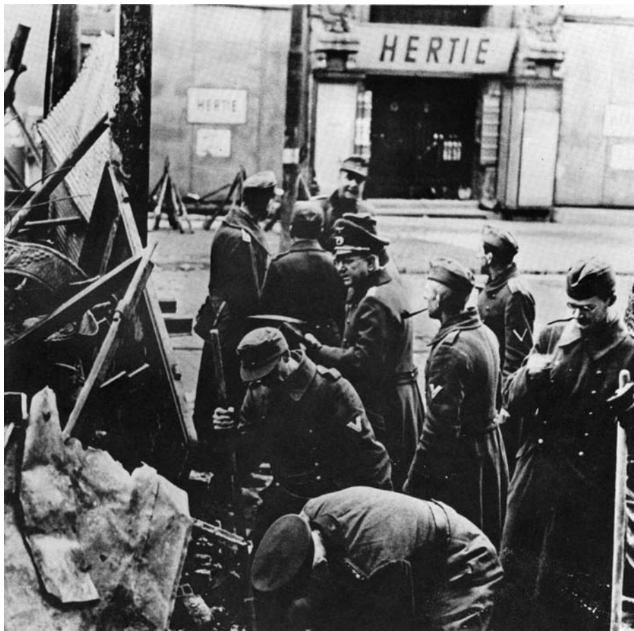
An officer directs German soldiers as they construct a barricade across a Berlin thoroughfare.
