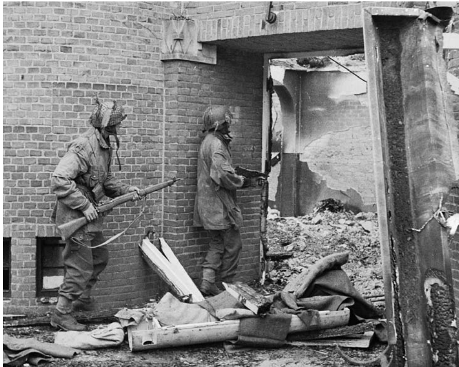
ABOVE: On September 20, 1944, NCOs of the Glider Pilot Regiment search for German snipers through the ruins of the ULO school in Oosterbeek, a town near Arnhem. An empty supply container lies just outside the shattered doorway. OPPOSITE: Firing his Enfield No. 2 revolver at the Germans from the window of the Hartenstein Hotel in Oosterbeek, headquarters of the 1st Airborne Division, a British para has sighted advancing Germans on September 23, 1944.
