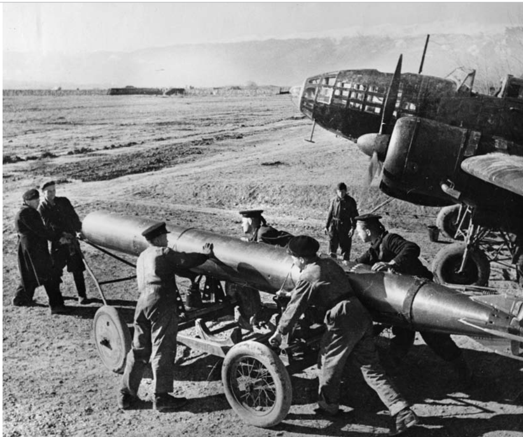
Soviet ground crewmen load a torpedo onto the versatile Ilyushin Il-4 twin-engined bomber. The Il-4 served as the backbone of the Soviet bomber corps throughout World War II.
