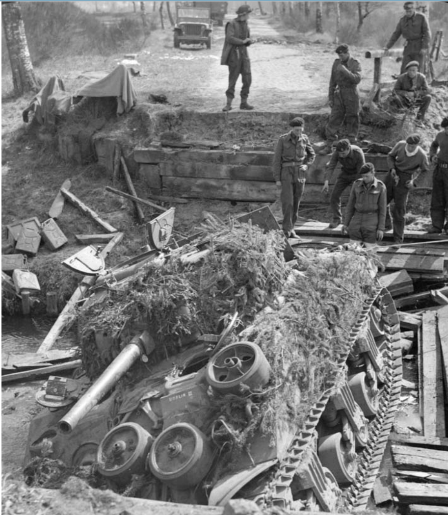
During the 21st Army Group drive toward the German city of Bremen, this Sherman tank attempted to cross a stream on an unstable bridge and collapsed it in the process. Armored vehicles that followed were compelled to seek another crossing point.
