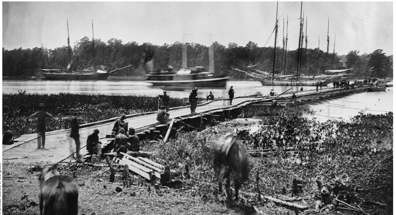
— — — — — Timothy O'Sullivan photographed the massive Union pontoon bridge over the James River at Weyanoke Point. Anchoring schooners can be seen in the background.
