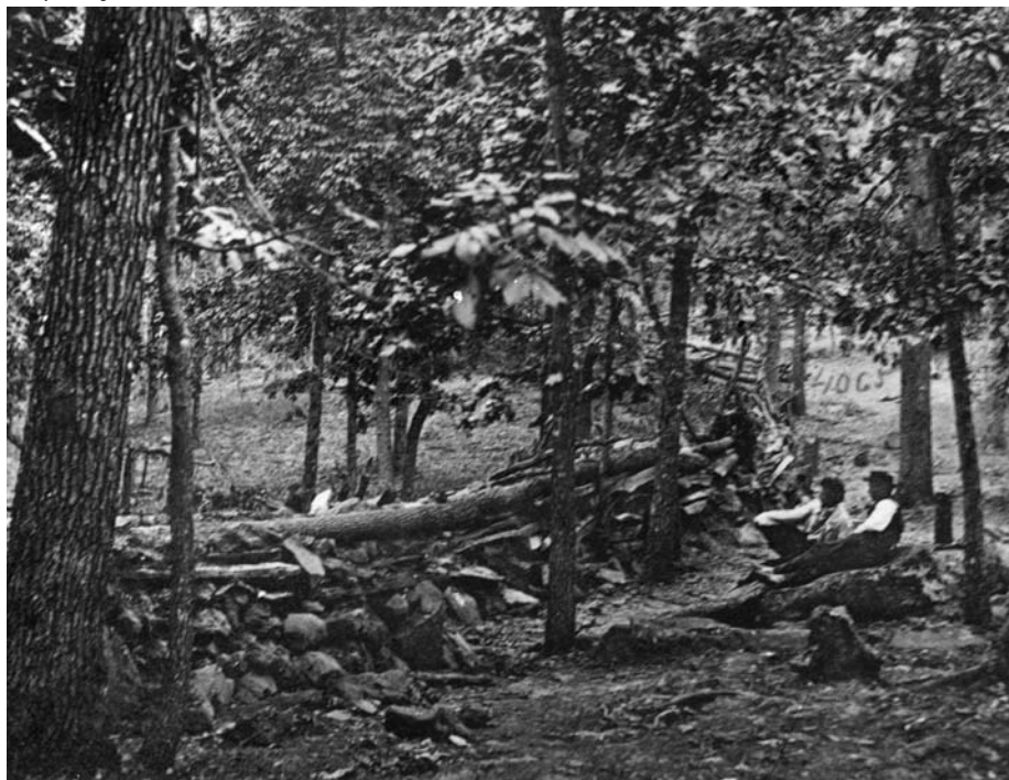
A photo taken after the battle testifies to the strength of the Union position atop Culp's Hill. The Yankees used rocks and logs to construct formidable breastworks.
