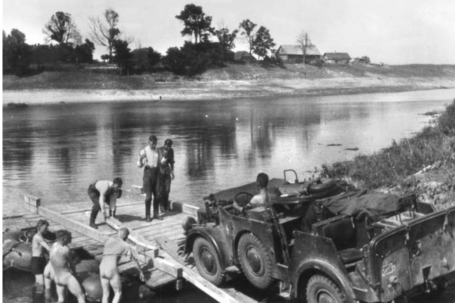
German engineers construct a bridge across a stream somewhere in the Ukraine during their advance in the summer of 1941. The engineers were also experienced combat troops.
