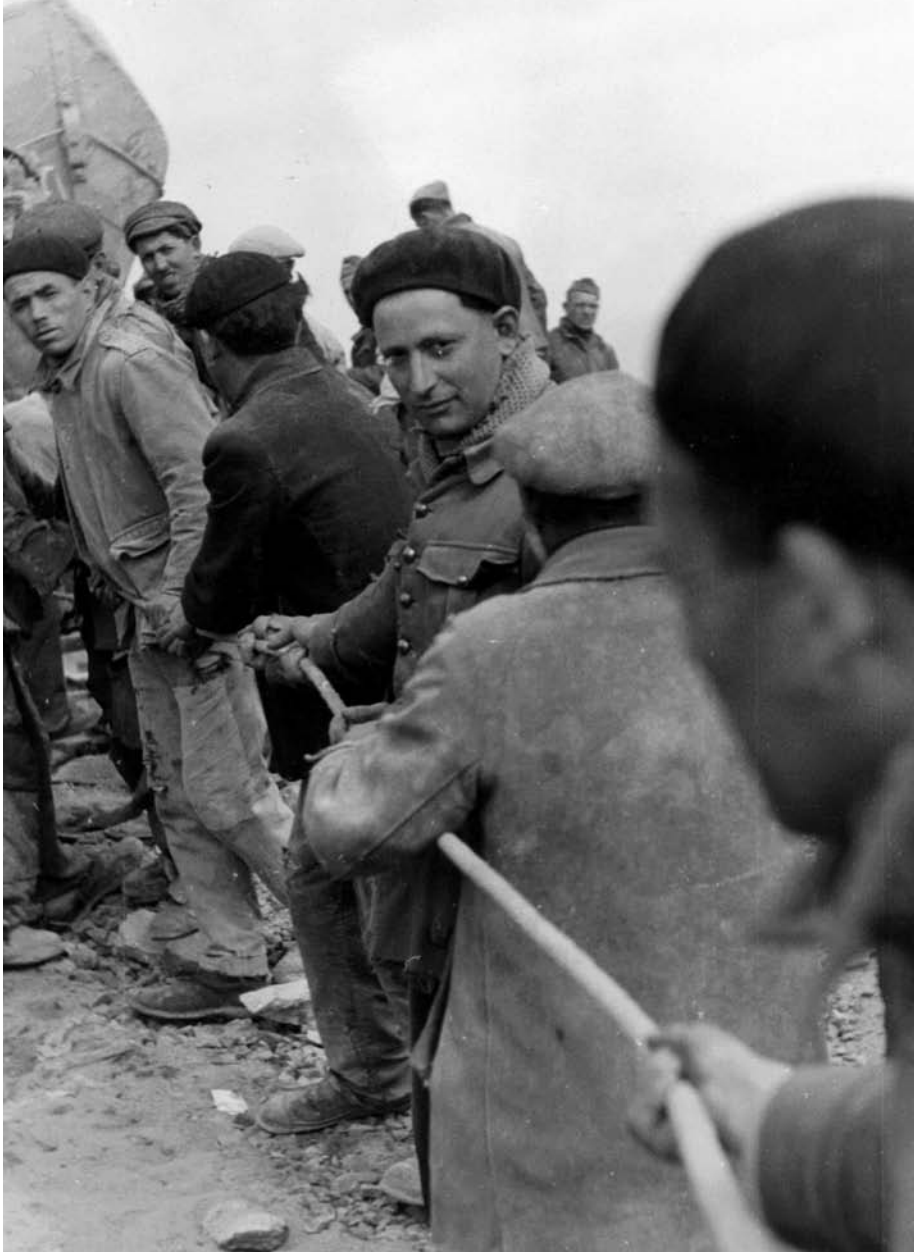
ABOVE: Not all the workers were willing. Here, conscripted laborers from a German-occupied country are put to work in May 1942. OPPOSITE TOP: More than a quarter million foreign workers, such as these Turks tying together reinforcing steel bars, provided much of the manpower to construct the fortifications. OPPOSITE BOTTOM: Dr. Fritz Todt (left) and Albert Speer supervised construction of the Atlantic Wall. Todt died in a mysterious plane explosion on February 8, 1942.
