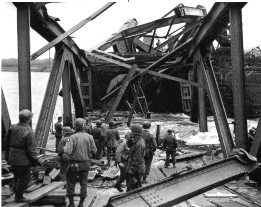
A mass of twisted steel is all that is left of the bridge when it fell into the river on March 17, killing 28 Americans.
