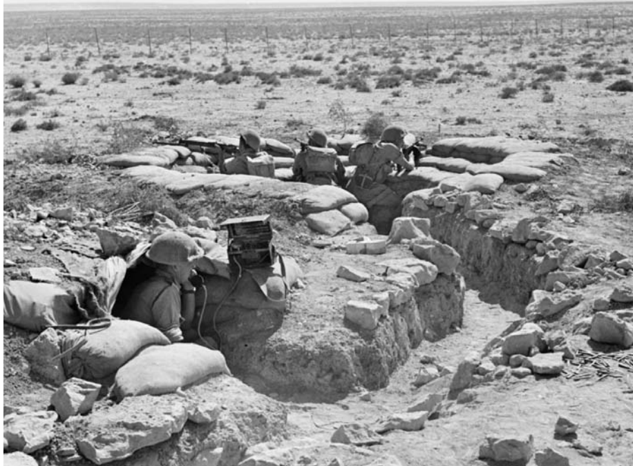
Australian soldiers man a strongpoint during the siege. These partly concealed, roofless pillboxes were located about every 1,000 feet around the perimeter. RIGHT: Australian troops march along the bottom of an antitank ditch, which the Italians had dug when they possessed Tobruk. OPPOSITE: An aerial photo of a key strongpoint in the southern sector of the Tobruk defenses reveals the strength of the network of defenses that enabled the Australians to repulse Rommel's elite units.
