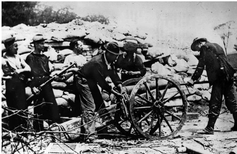
ABOVE: U.S. Marines man an improvised cannon assembled from a Chinese tube, British trail, and Austrian carriage wheels. The gun fired Russian and Chinese shells. RIGHT: Although a large number of American troops were tied up fighting the Philippine Insurrection, 1,300 men of the 9th Infantry began arriving in Tientsin on July 11, 1900. A detachment is shown manning a Gatling gun.
