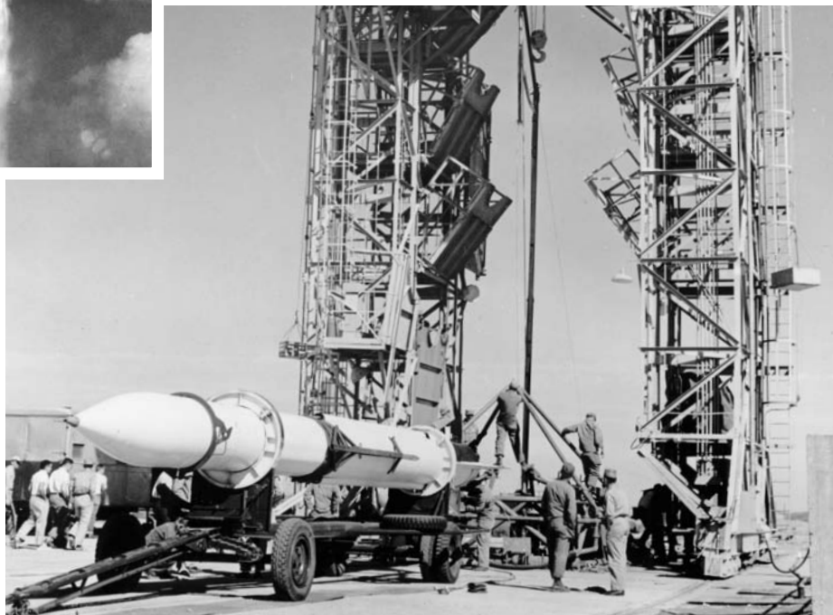
LEFT: WAC "baby" Corporal loaded atop a German V-2 rocket for testing at White Sands Proving Ground, New Mexico, in 1949. BELOW: Corporal Model E being prepared for loading at White Sands Proving Ground on August 3, 1951.
