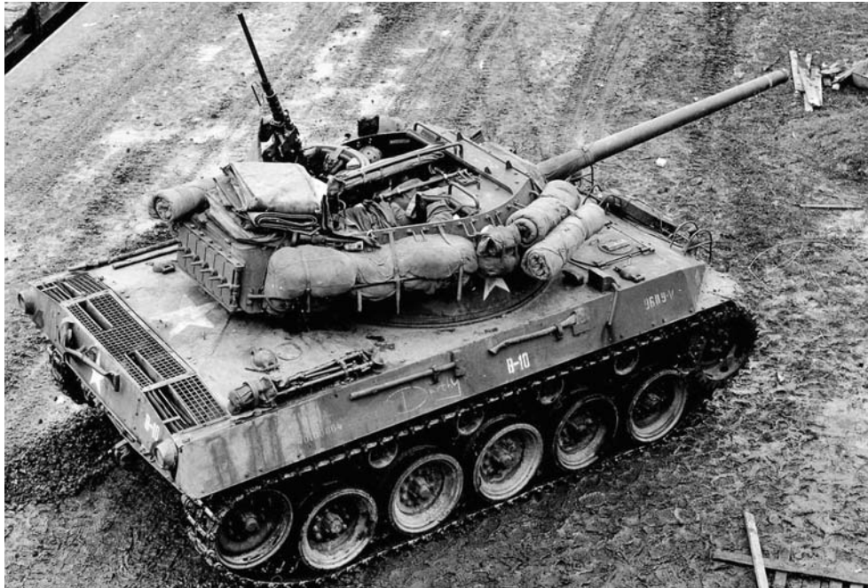
ABOVE: One of the major drawbacks of the open-turret M18 was that its 76 mm gun was little better than the 3-inch gun of the M10. Moreover, many tank destroyer crews preferred the configuration of the M10's fighting compartment. BELOW: M18 Hellcat crews, such as this one the Ardennes in December 1944, reported that their vehicles could go hundreds of miles under trying conditions without requiring major repairs to the armaments or the engine.
