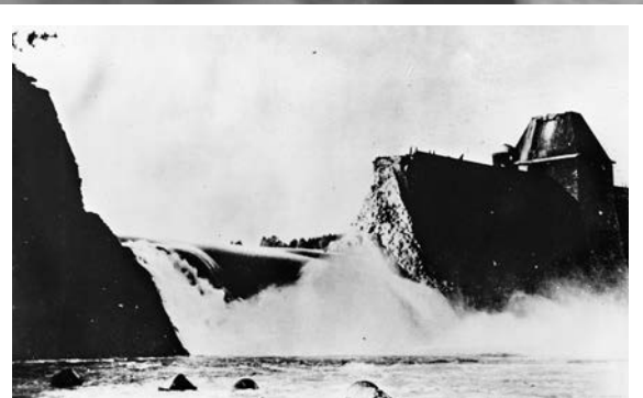
ABOVE: Most of the 30 billion gallons of water impounded by the Möhne Dam is gone in this aerial reconnaissance photo taken by a Spitfire Mk. XI on May 17, 1943, the morning after the RAF Dambusters raid tore a roughly 250-foot-square hole in the structure. INSET: Closeup of the breach of Germany's Möhne Dam on May 17, 1943, some 4.5 hours after the Operation Chastise raid. OPPOSITE: Contemporaneous illustration of modified Lancaster bombers on the daring "Dambusters" raid of May 16-17, 1943, that so captured the public's imagination.
