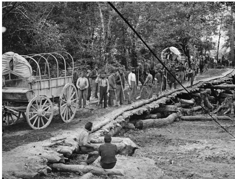
Members of the 5th New Hampshire Infantry admire their work on the hastily constructed Grapevine Bridge across the Chickahominy River at Seven Pines. The rough bridge was crucial to funneling reinforcements to the battlefield.
