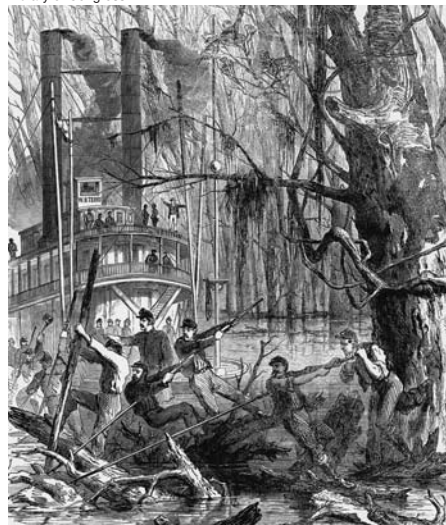
ABOVE: Federal engineers break up a log jam in Wilson's Bayou. OPPOSITE: A Union floating battery lets loose with a massive blast from its 32-pounder mortar.
