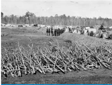
ABOVE: Abatis made of tree limbs can be seen in the foreground as part of the fortifications at Fort Brady on the James River. RIGHT: The breastworks at Fort Mahone, Petersburg, are seen in this 1865 photo. RIGHT BOTTOM: Federal troops occupy a line of simple breastworks on the north bank of the North Anna River in Virginia.
