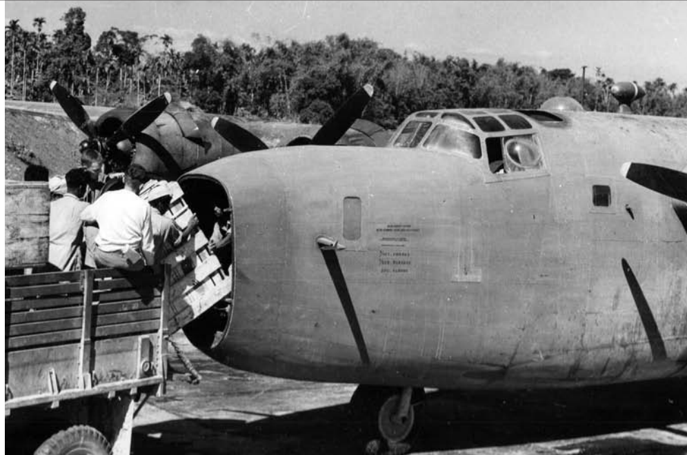
ABOVE: Men transfer naval stores from a truck into the nose of a Consolidated C-87 for shipment to China. The nose of this plane provides cargo space for three drums of gasoline and a 500-pound bomb or its equivalent. RIGHT: Major Louis E. Scherck, Houston, Texas, 40th Bomb Group, XX Bomber Command in China, “pitches in” and rolls empty gasoline drums to trucks waiting to haul them to another area. OPPOSITE: Curtiss C-46 Commando in the snow-capped Himalayas between India and China. Every two and a half minutes, the India-China Division of ATC puts a plane across this route.
