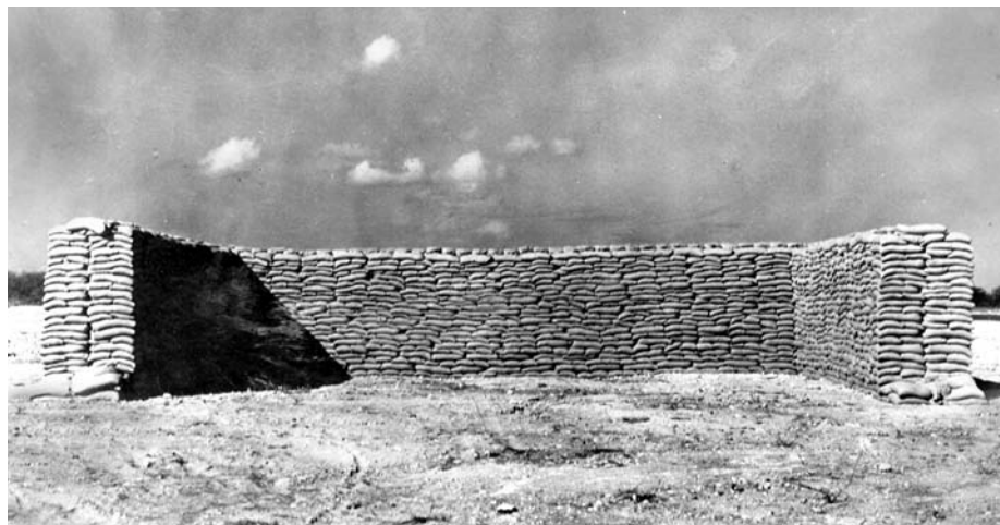
ABOVE: The Marines at Ewa had constructed numerous sandbag revetments for the protection of parked aircraft before December 7. However, many planes were parked in the open on the morning of the fateful attack due to fears of sabotage. TOP: As the focus of Ewa Marine Corps Air Station changed from airships to military aircraft operation, the dirigible mooring mast was converted into a control tower, as shown in this February 1941 image. OPPOSITE, TOP: Planes at Ewa Marine Corps Air Station in early 1941, including four Grumman F3F-2 biplane fighters of Marine Fighting Squadron-2 (VMF-2), 13 Douglas SBD-1 Dauntless dive bombers of Marine Bombing Squadron-2 (VMB-2), and other planes.
